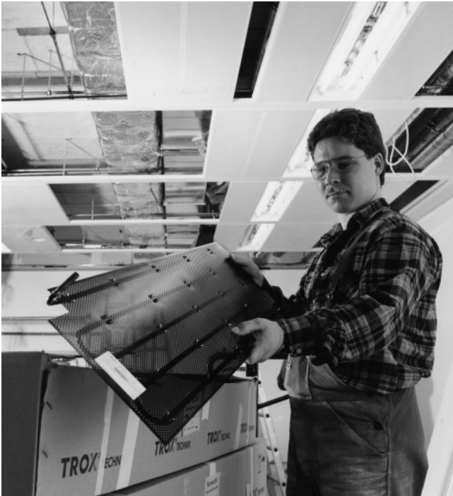
Figure 1: Mounting of WK-D-UM
