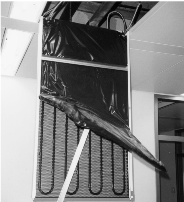
Figure 2: Hinged chilled ceiling with ceiling cooling element type WK-D-UM (e. g. for inspection)
