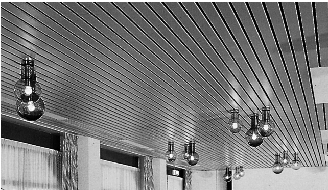
Figure 6: Chilled panel ceiling
