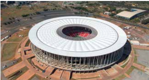
Estádio Nacional, Brasília: TROX ventilation and air conditioning in all newly built World Cup stadia in Brazil
