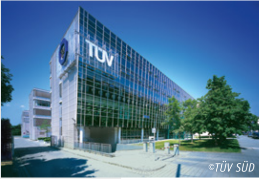
TROX air handling units are regularly examined (e.g. by TÜV SÜD, Germany)
