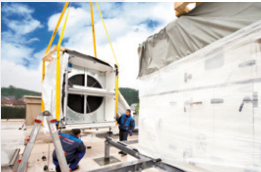
Delivery and installation of a weatherproof X-CUBE
