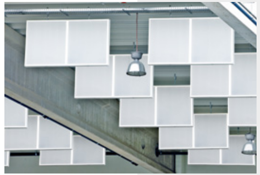
Optimised plant acoustics thanks to TROX splitters
